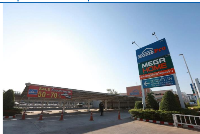
Figure 3: HomePro and Mega Home stores in the same compound in Khon Kaen province
